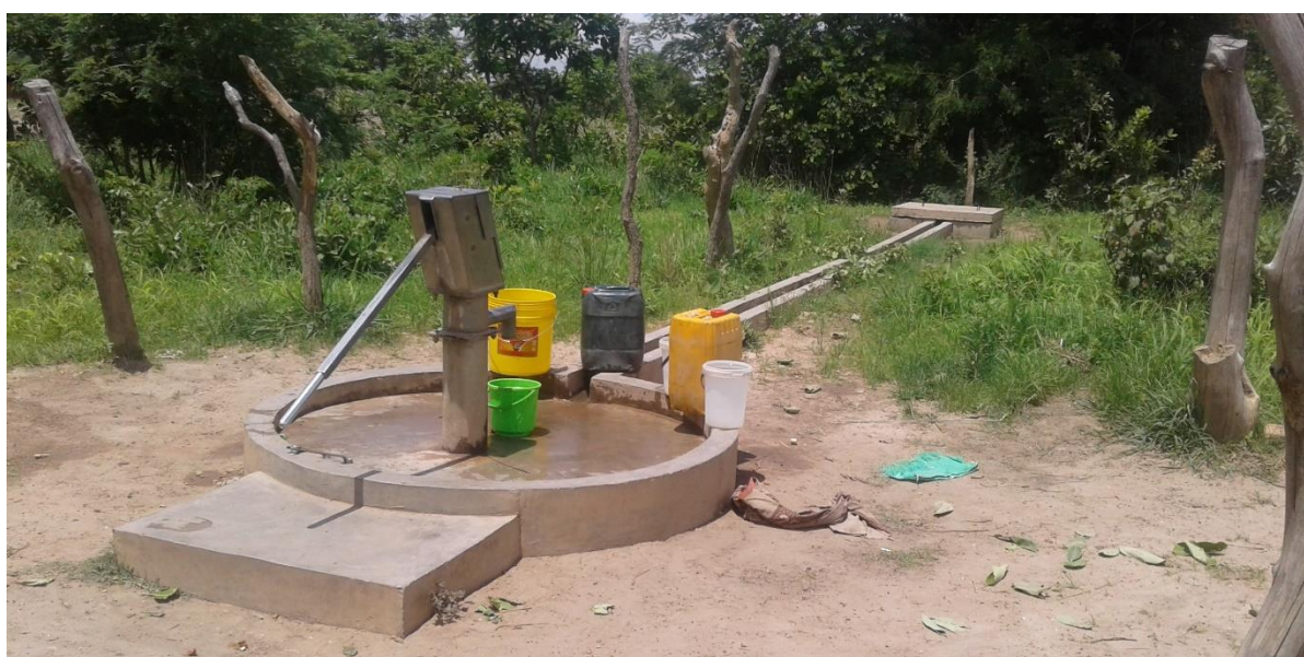
Picture 5: Ghana Modified India Mark II hand pump, Chongwe
