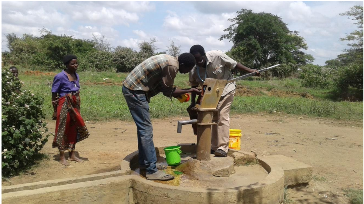
Picture 3: Applying grease to chain on hand pump at Nkomeshya Village, Chongwe
