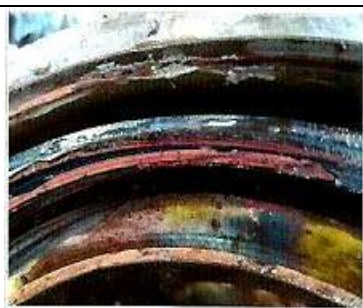
Brake Seal With Silastic Sealing
