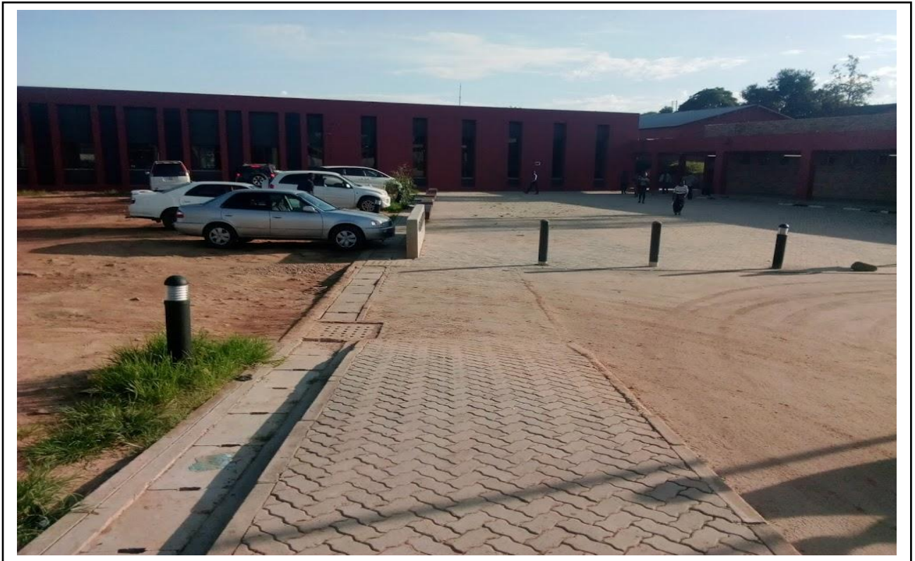
Figure 4: Matero First Level Hospital (ZANIS, 2020).
