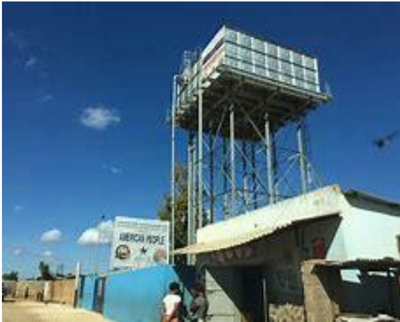
Figure 4.2: water tank. (source: field survey, 2025)
