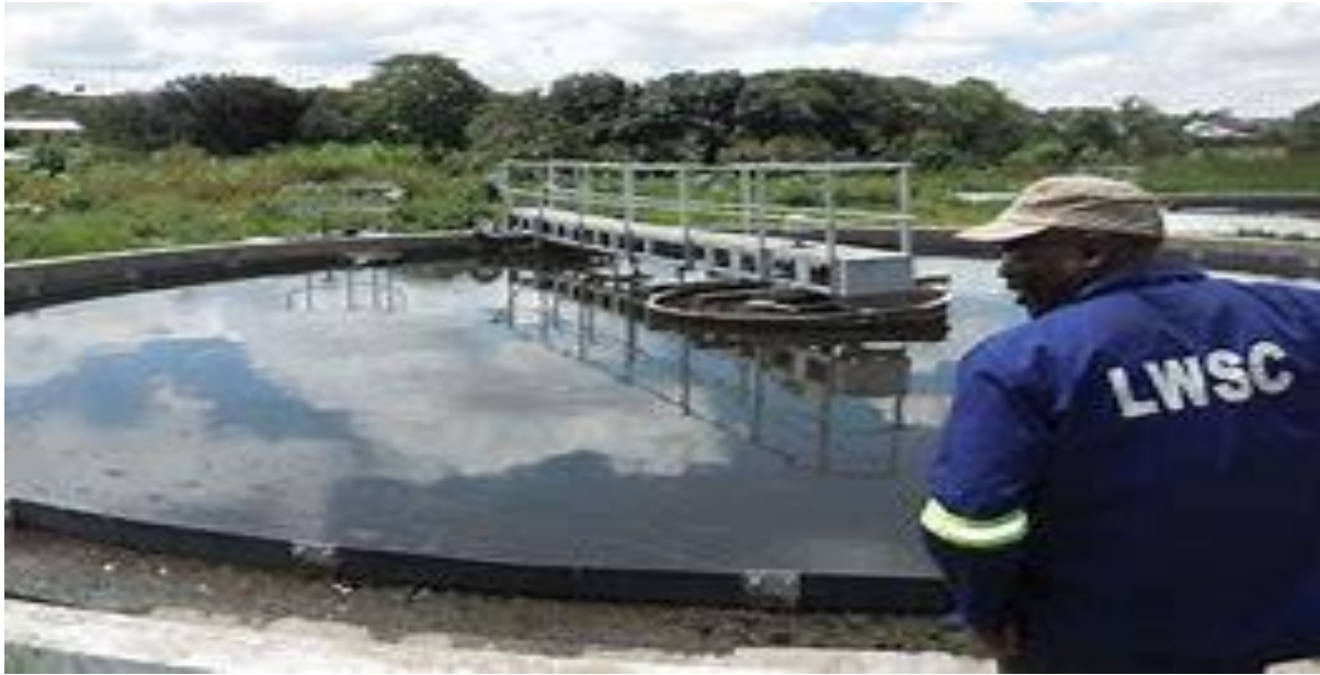
Figure 4.1: water plant. (source: field survey, 2024)
