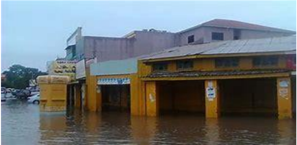
Figure 1.1: Floods as a results of improper drainage system or clogged drainages. Source: (LWSSC website).
