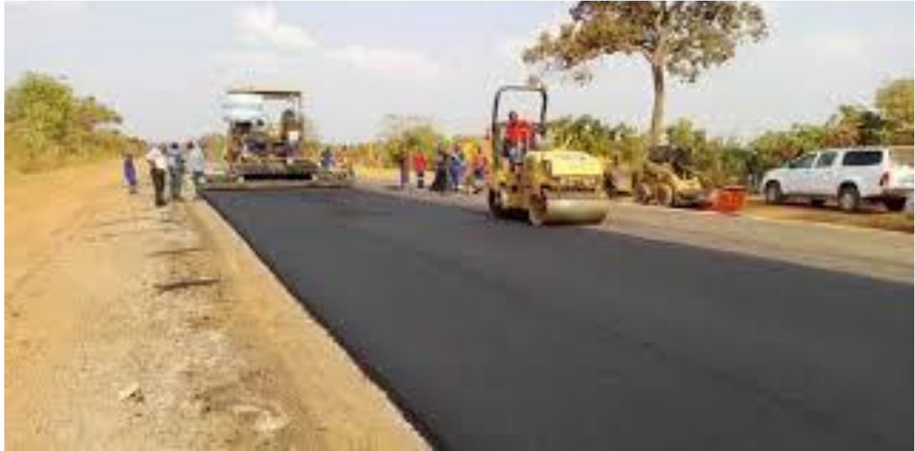
Figure 6: Newly built Chingola Solwezi road
