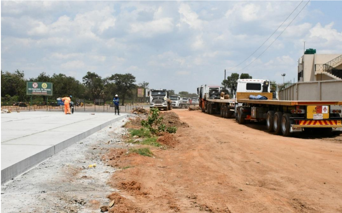
Figure 1: Newly built Lusaka Ndola carriage way in Ndola Researcher (2023)
