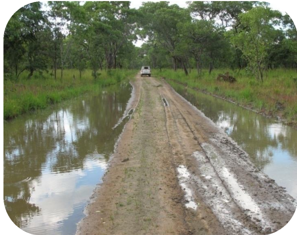
Figure 61: Flooded and Soft Spots on Spinal Road due to 2012-2013 rains
