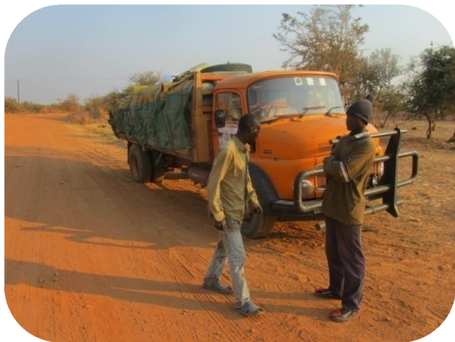
Figure 65: Deteriorated Nyawa road in Zimba
