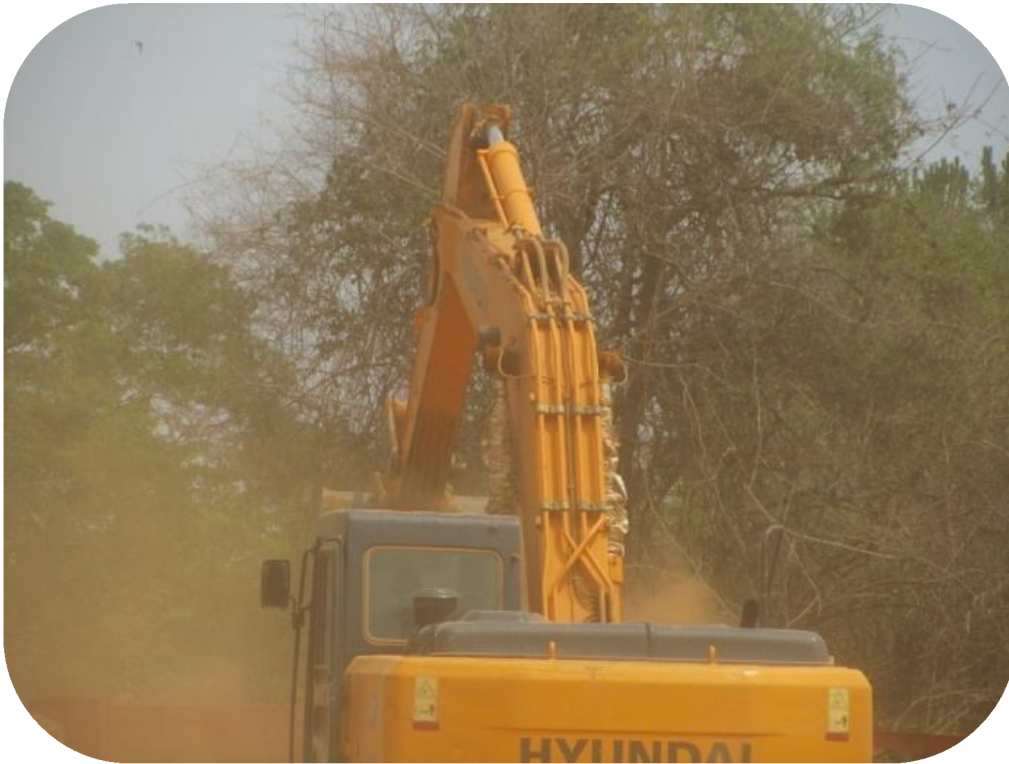
Figure 43: 2 nd Generation OPRC Contracts were successful due to good preparation and financing (D361 Road in Choma, 2010)
