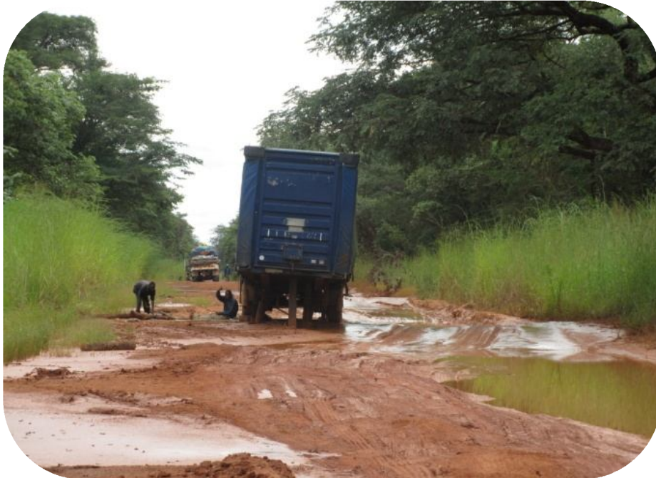
Figure 2: Deteriorated pedicle road (gravel road)
