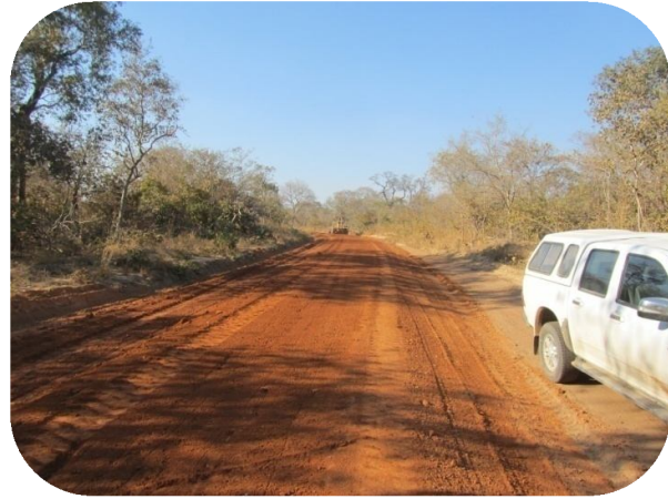
Figure 56: Works in Progress on Spinal Road
