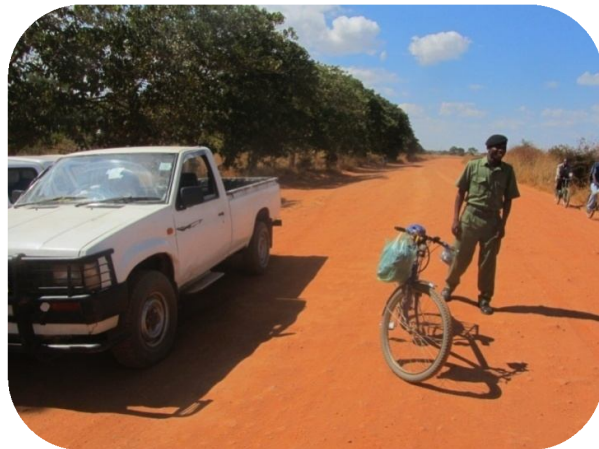
Figure 62: Deteriorated Monze – Niko Road after rehabilitation in 2010
