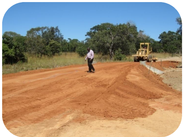
Figure 57: Researcher inspecting improvement works on Spinal Road
