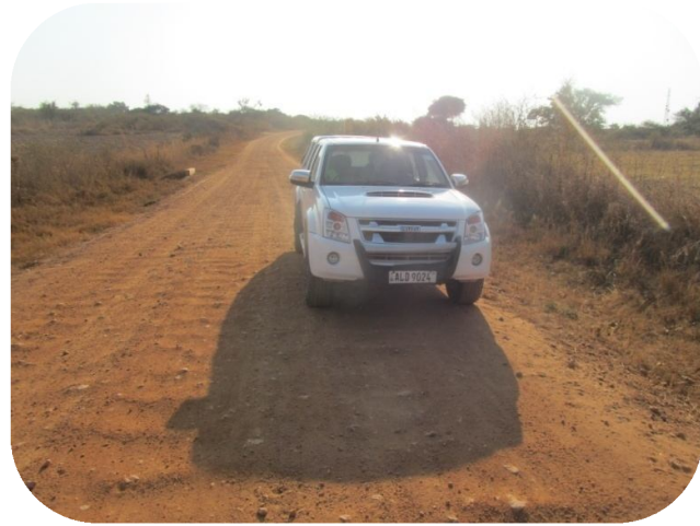
Figure 68: Corrugations on Ruyala road in Zimba
