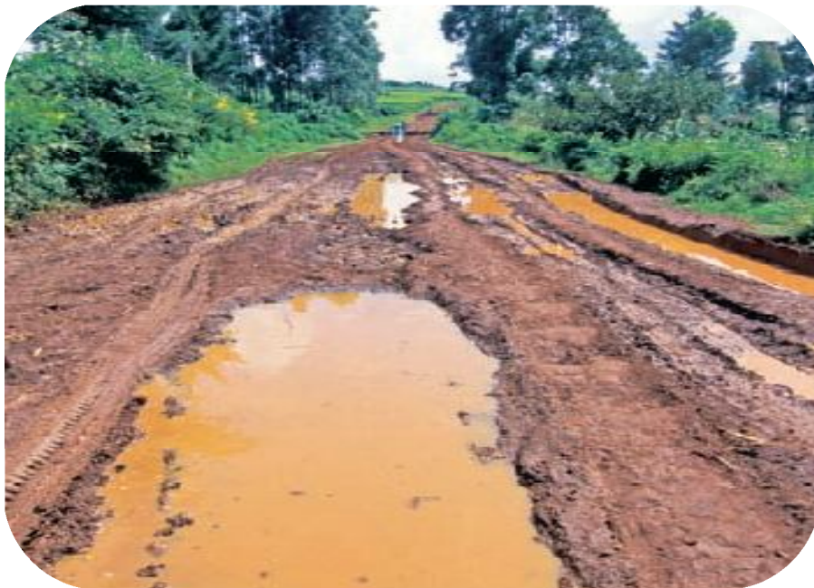
Figure 1: Typical condition of most gravel roads in the rainy season in Zambia
