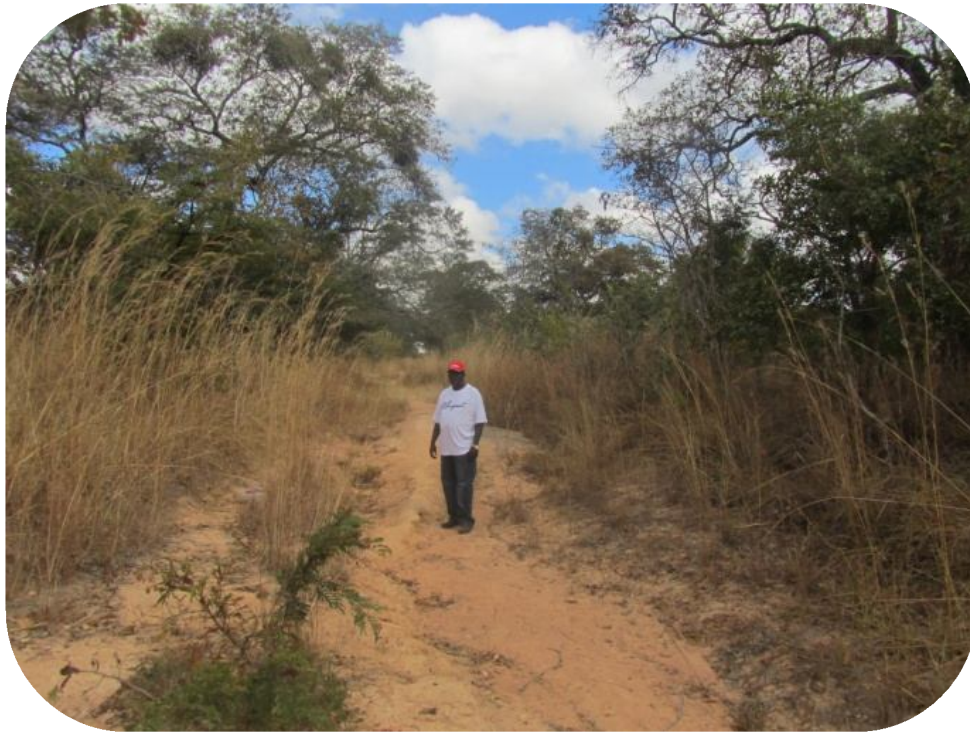
Figure 3: Most Gravel roads in Zambia have deteriorated due to lack of strategic maintenance ( Choma to Prison's farm road, 2013 )
