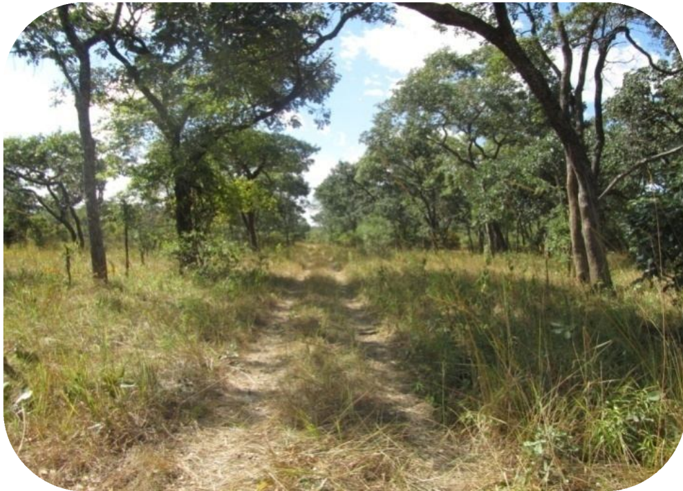
Figure 55: Spinal Road before Rehabilitation in KNP: the consequences of lack of Sustainable Road Maintenance System-A sign of non application of Lean Thinking and Value Management Philosophies
