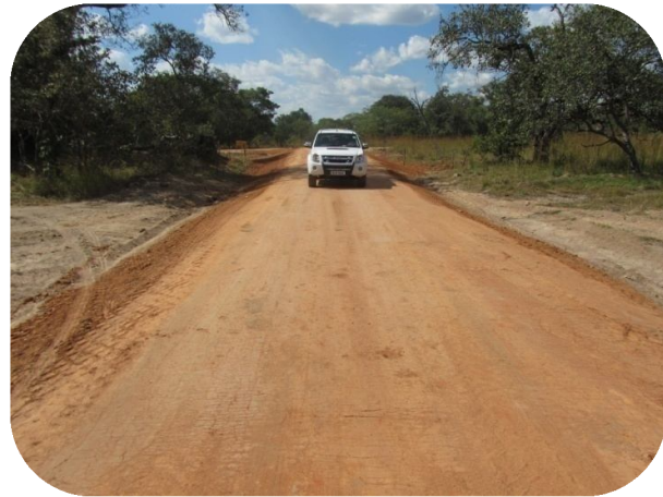
Figure 58: Rehabilitated Spinal Road in KNP
