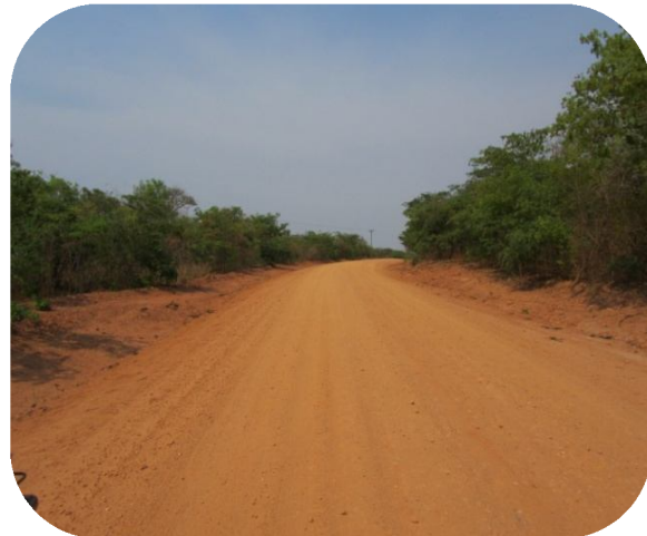
Figure 54: A road in Katete after improvement with OPRC
